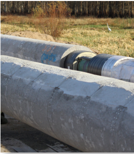
Optimized thermal insulation coated with 2.5" concrete to overcome buoyancy
